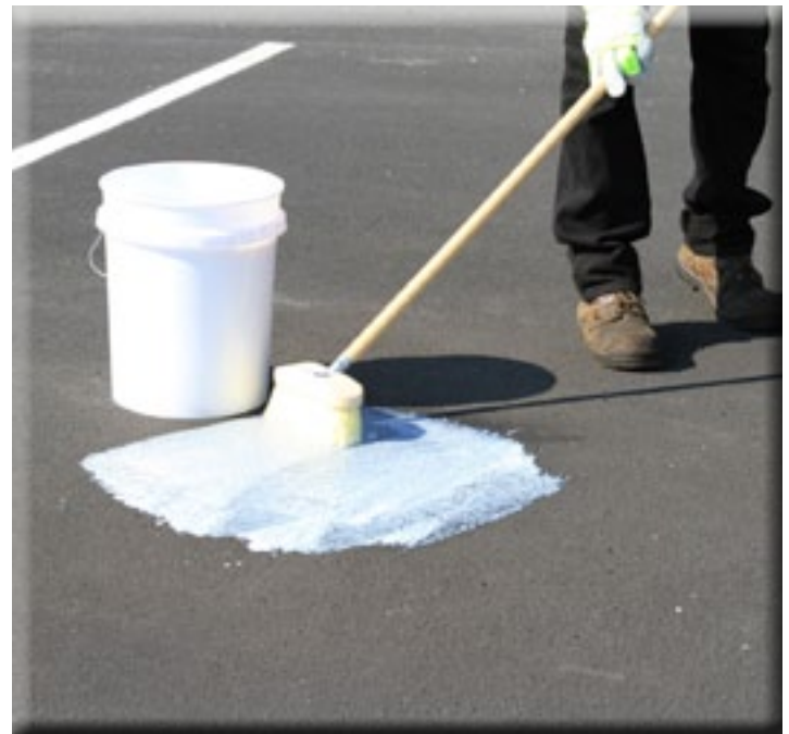
Applying SealMaster Oil Spot Primer
