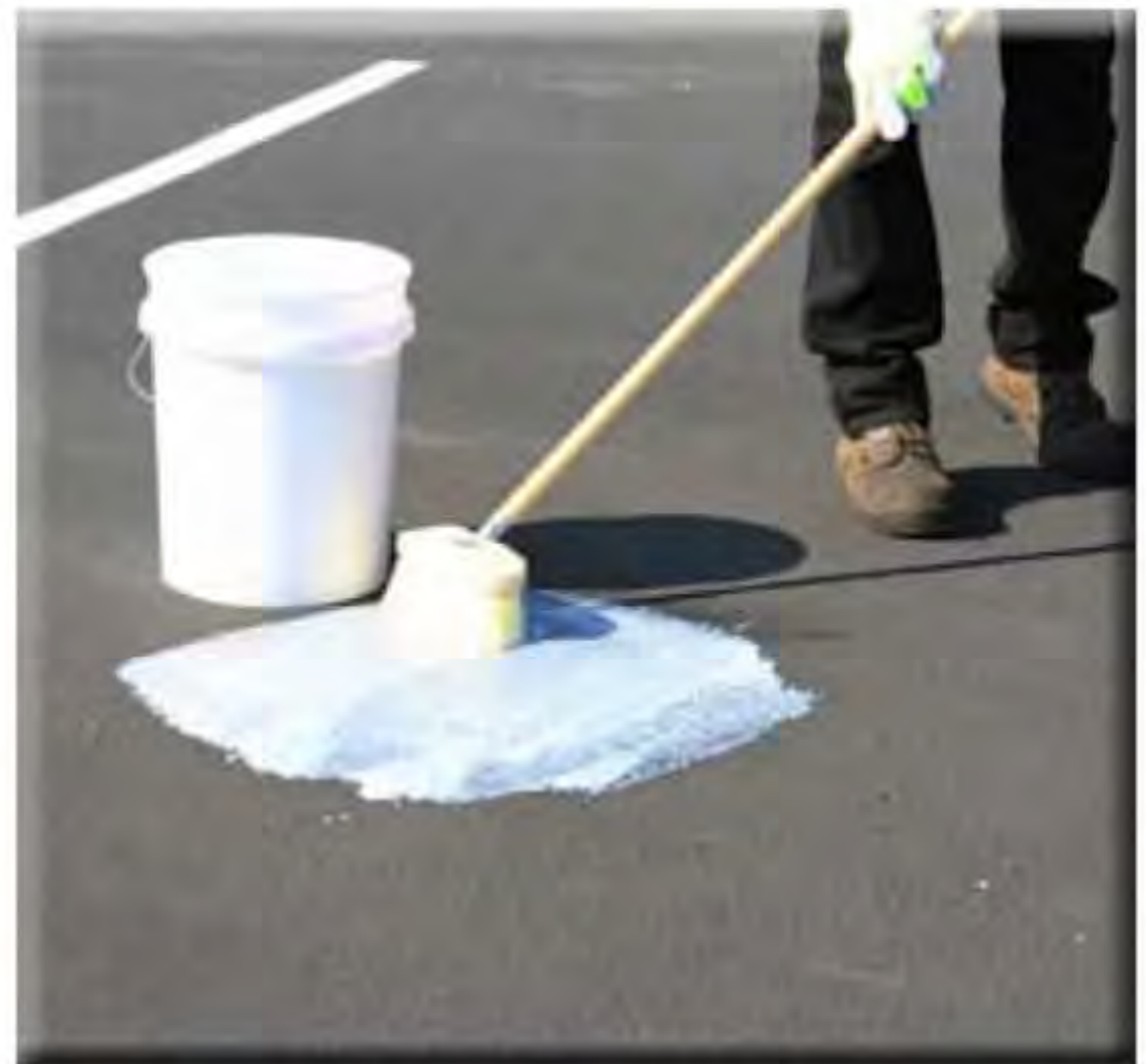
Applying SealMaster Oil Spot Primer
