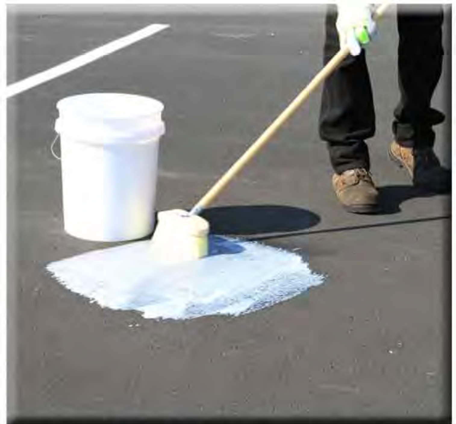
Applying SealMaster Oil Spot Primer
