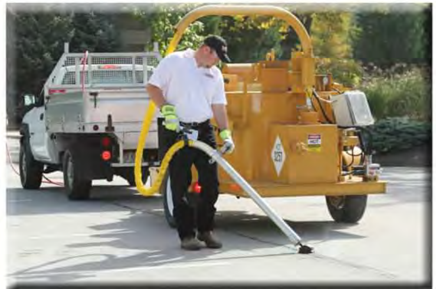
Crack Filling
