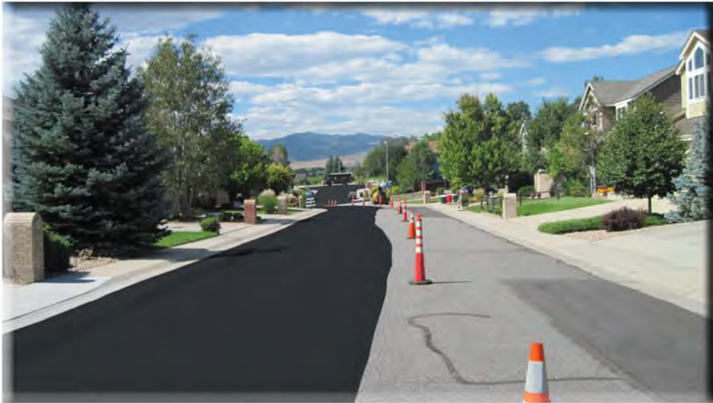
Left side shows application of Liquid Road® Bituminous Surface Treatment
