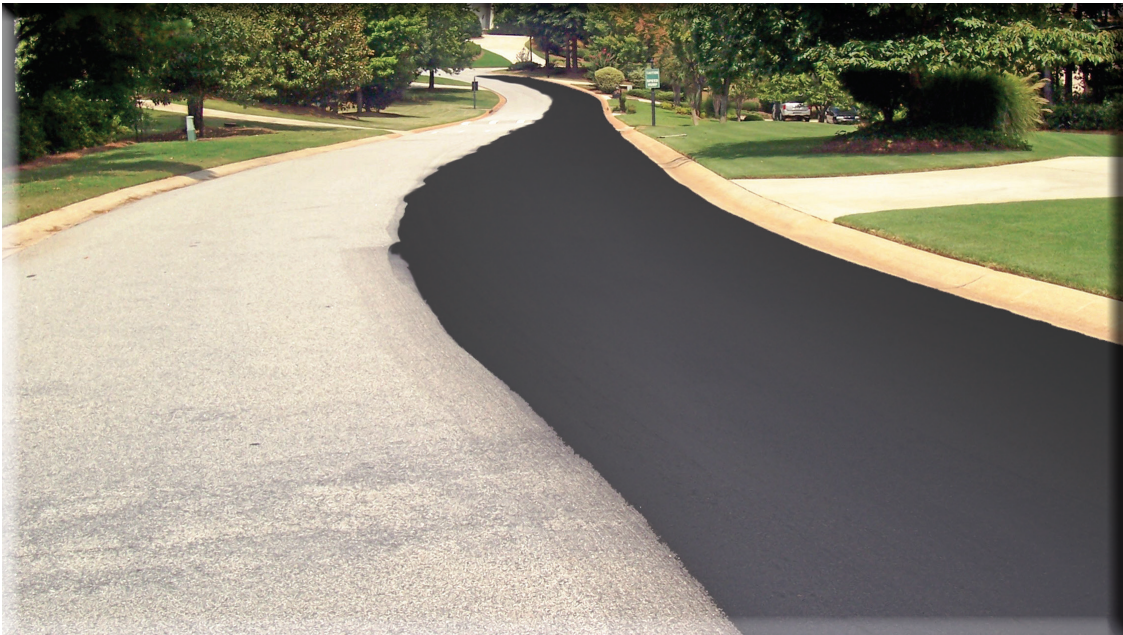
Right side shows application of AsPen® Surface Sealer
