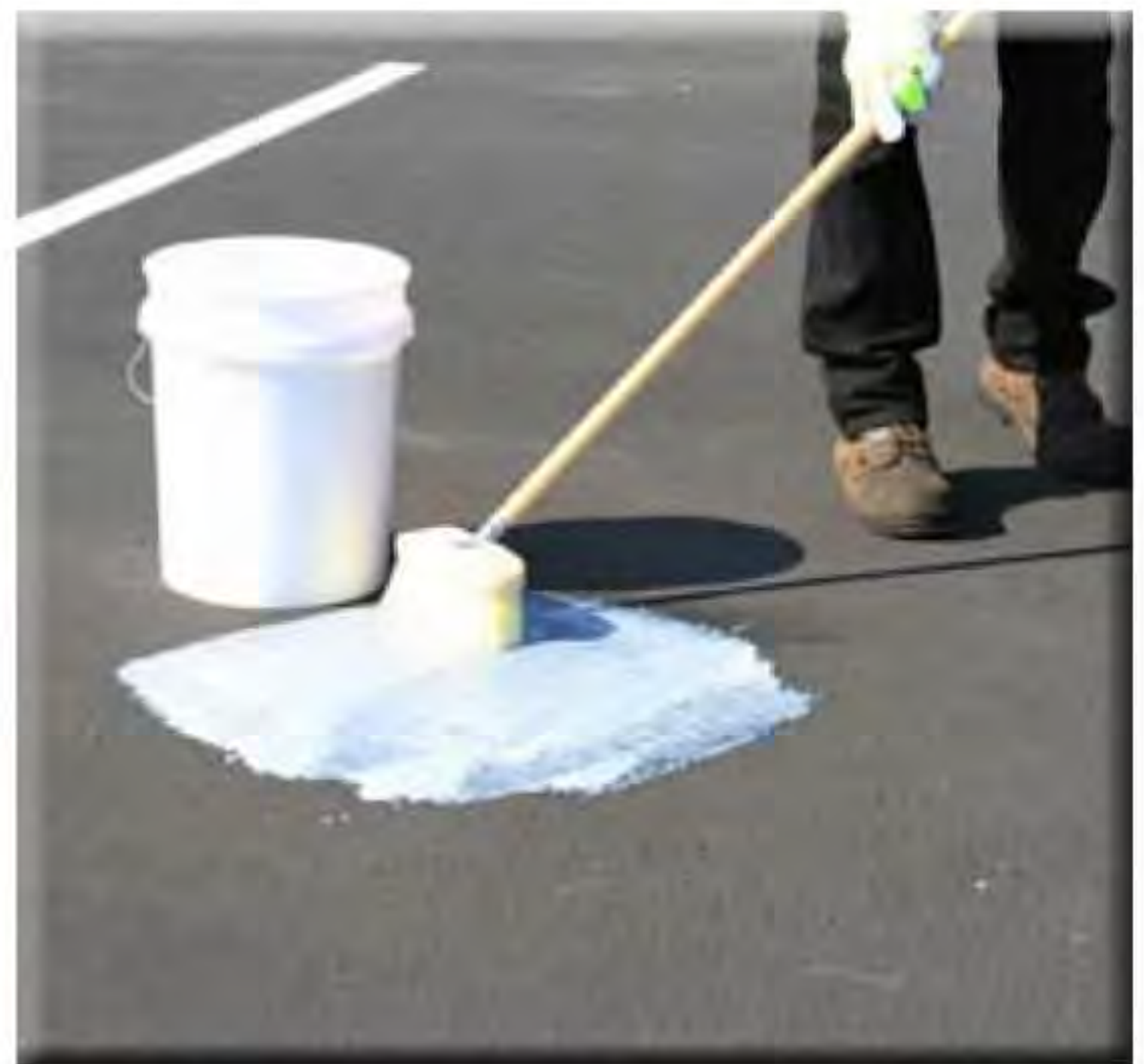
Applying SealMaster Oil Spot Primer
