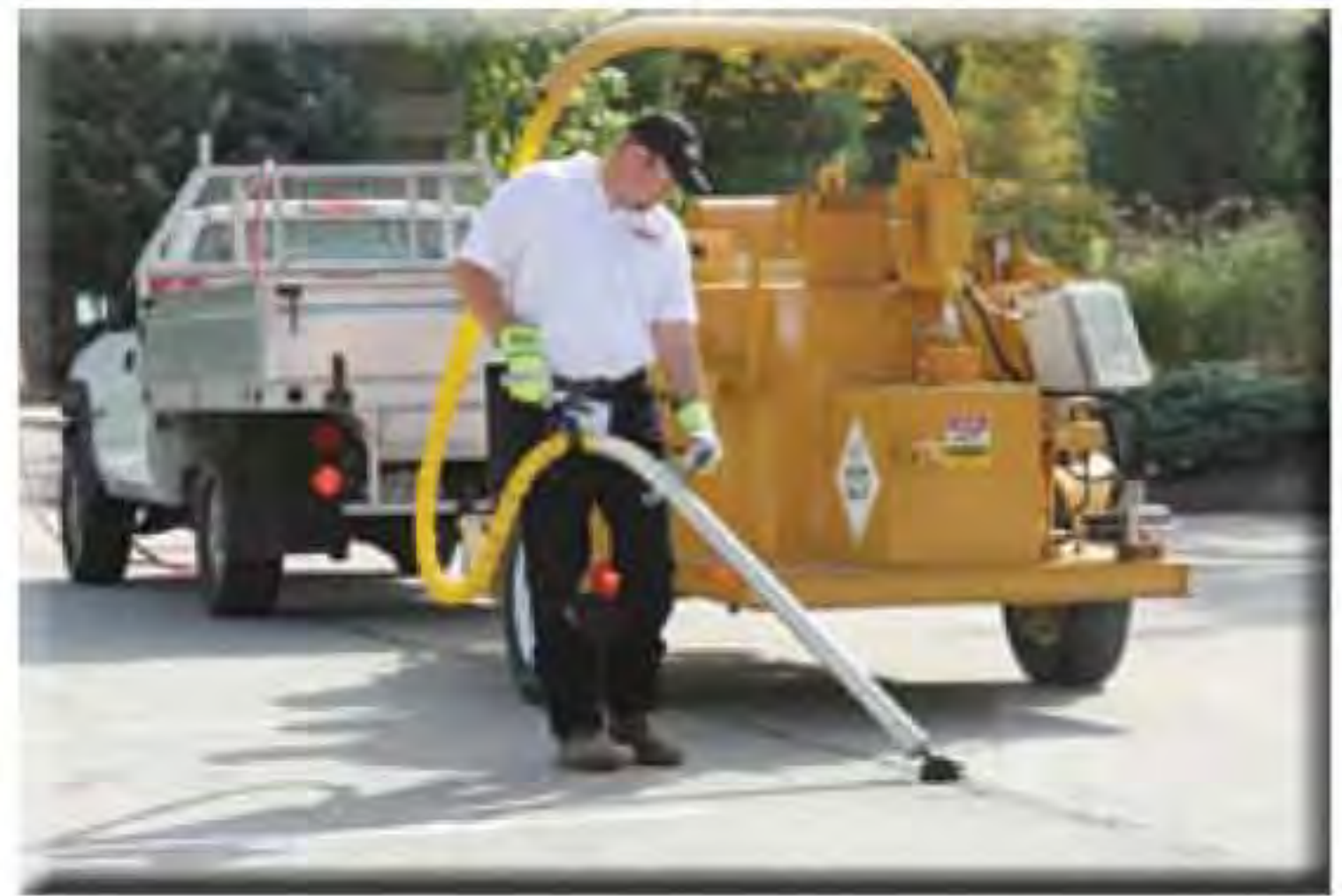
Crack Filling
