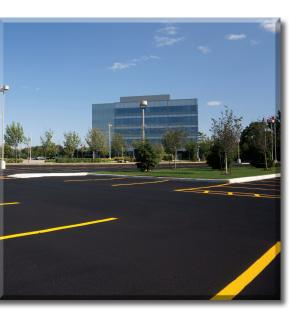
A pavement maintenance program that includes periodic sealcoating and crack filling will more than double the service life of asphalt pavement.
