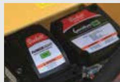
Diesel fired Beckett Burner
